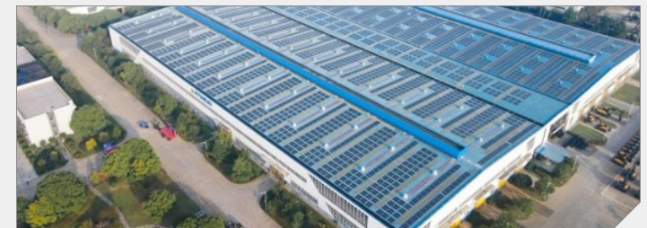
Solar power generation on the rooftop for the Chinese subsidiary (4 MW)
